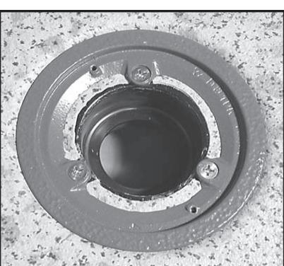
11) Install retainer clamping flange with (3) screws (supplied)
