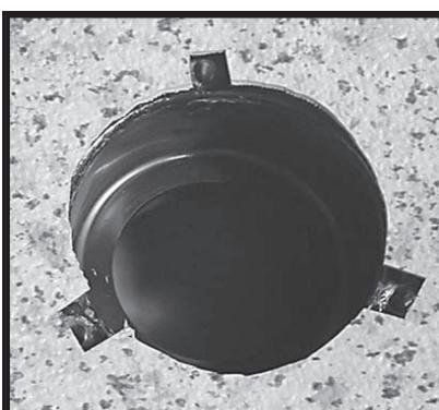
9) Install membrane, cut 3" dia hole (centered), cut patches at clamping flange fastening points
